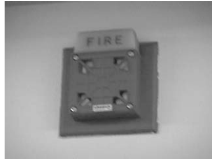
Figure 4.4. Horn and Strobe
