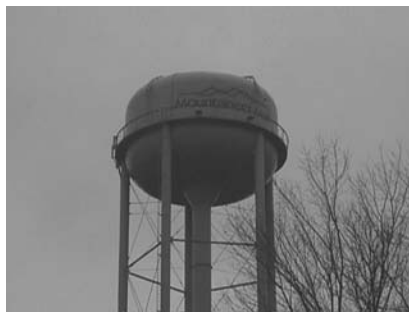
Figure 4.10. Elevated Water Tank 2
