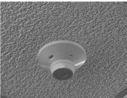
Figure 4.1. Smoke Detector
