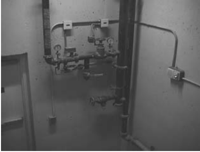
Figure 4.5. Stairwell Standpipe
