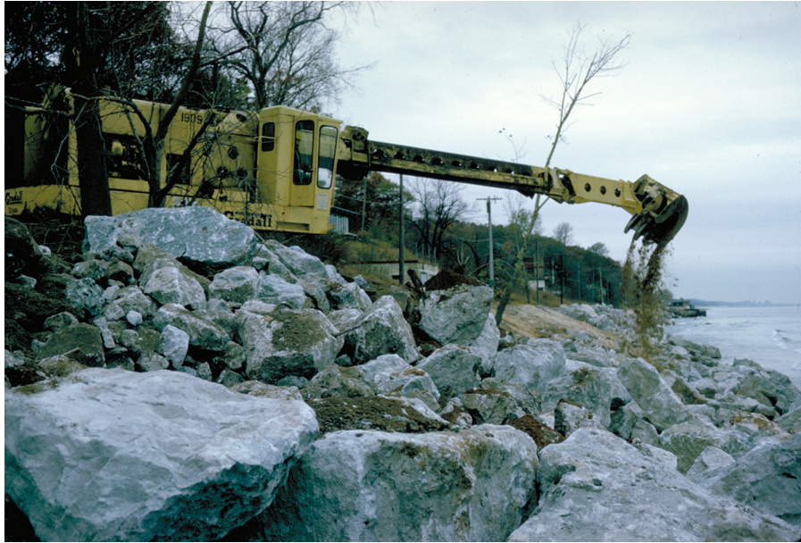
■ FIGURE 9.6 Shoreline revetment project in Indiana. Image by the National Park Service, Indiana Dunes National Lakeshore. Courtesy of EPA.
