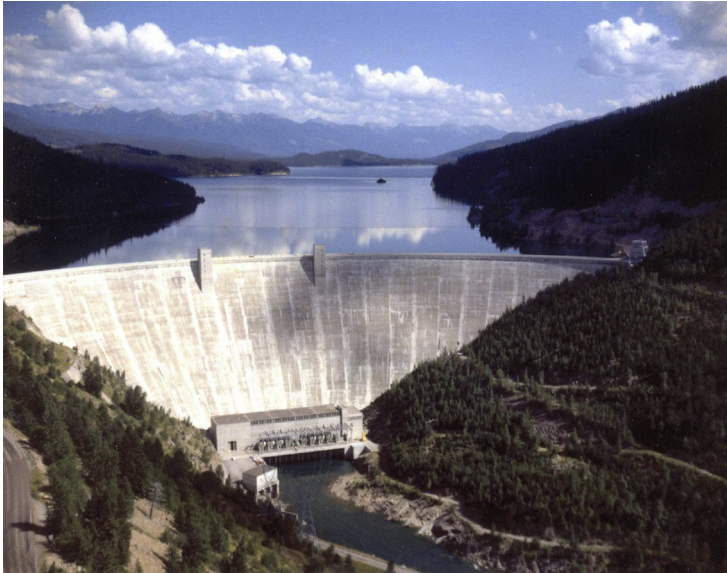
■ FIGURE 9.2 At 564 feet (172 m) high, Hungry Horse Dam in Montana is one of the largest concrete arch dams in the United States. Courtesy of the U.S. Bureau of Reclamation.
