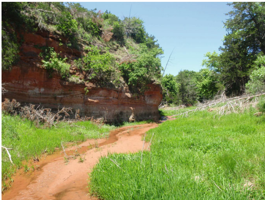
Fig. 5.1 A dam failure in sandy soil caused by intense and prolonged precipitation (breach is in background on right )
