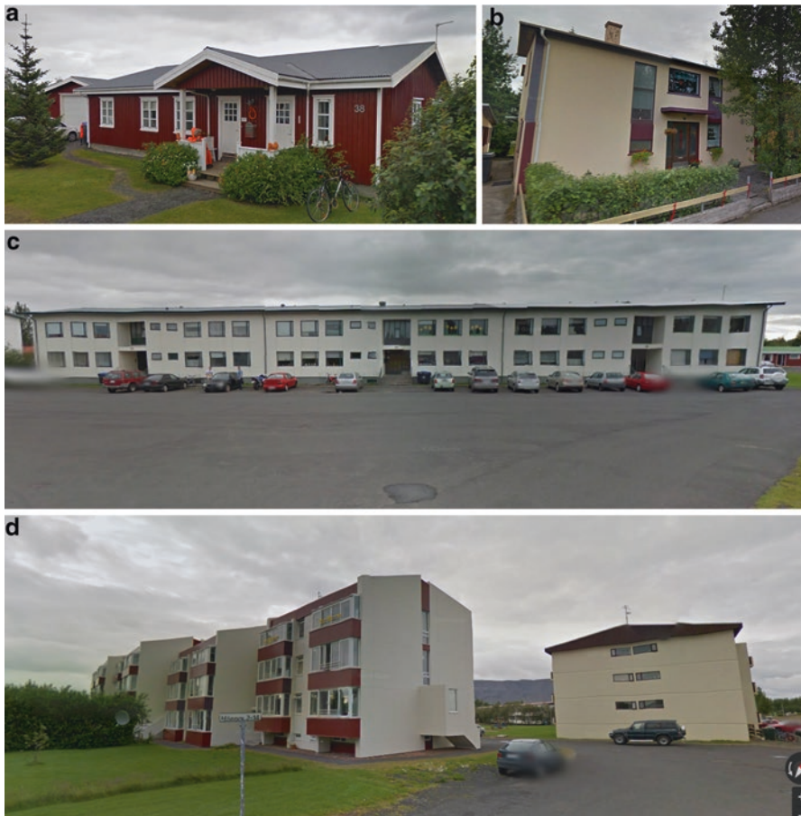
Fig. 11.7 Examples of buildings in the town of Selfoss in south Iceland: (a) single-story timber building; (b) two-story RC building; (c) two-story RC apartment block; (d) three-story RC apartment blocks (Google maps – Street viewer)
