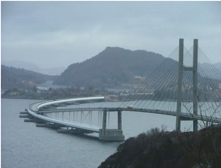
Fig. 15.1 The Nordhordaland Bridge with floating pontoons (located at the west coast of Norway)
