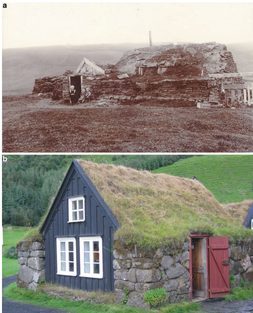
Fig. 11.3 Turf and stone houses: (a) from Húsavík around 1900 (Photo: Icelandic and Faroese Photographs of Frederick W. W. Howell, Cornell University Library), (b) from Skógar Museum in south Iceland
