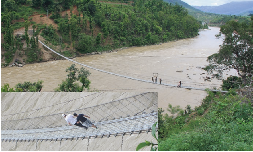
Fig. 10 Main photo: The Abu Khairini Suspension Bridge over the Marsyangdi River in Gorkha, Nepal inset: Ragnar with Rajesh following him, crossing the bridge and investigating its vibrational characteristics
