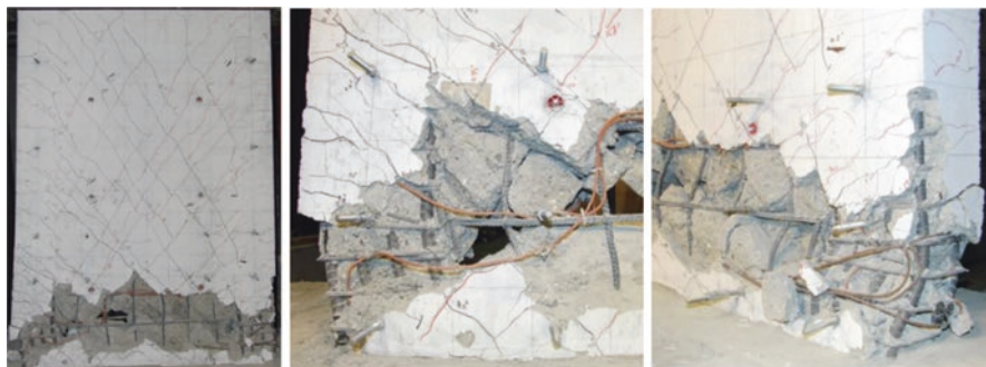
Fig. 5.10 Damage of the specimen RW-A15-P10-S78 after the test (Tran and Wallace 2012)
