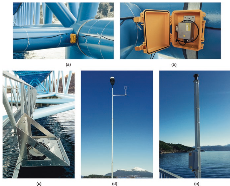
Fig. 14.8 Sensor photos: (a) triaxial accelerometer with closed enclosure, (b) accelerometer with open enclosure, (c) wave radar, (d) anemometer in lamp post, (e) GNSS sensor in pole (Reprinted from Kvåle and Øiseth (2017), with permission from Elsevier)
