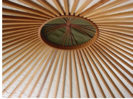
Wooden structure (frame) of a yurt
